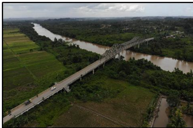
Figure 2. Aerial photo of the old Kutai bridge
